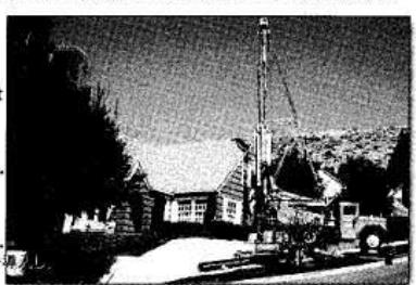
A drilling rig sets up to install underground pipes for a geothermal heat pump going into this home in Klamath Falls, Ore.
